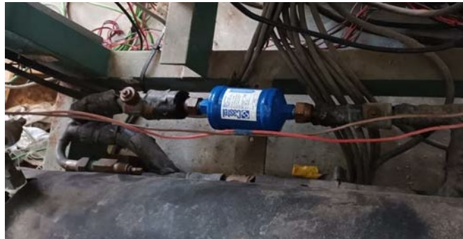
Figure 4. Filter installed for testing
